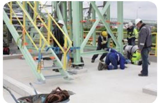
Reducing alignment time on site
