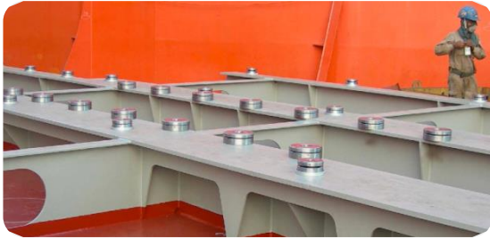
Preparation of compressor set chocking
